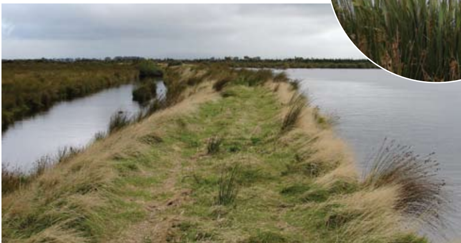
The track in the centre of the image follows the artificial dam that allowed the lagoon on the right to fill again. On the left, a portion of the ring drain is visible; note that the level of the lagoon is raised some distance above the drain.
